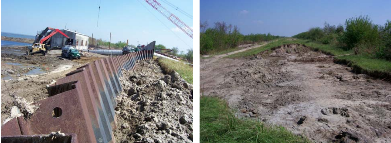
FIGURE 2. Damage at Pump Station 15 (left) and to LPV 111 levee (right), following Hurricane Katrina
